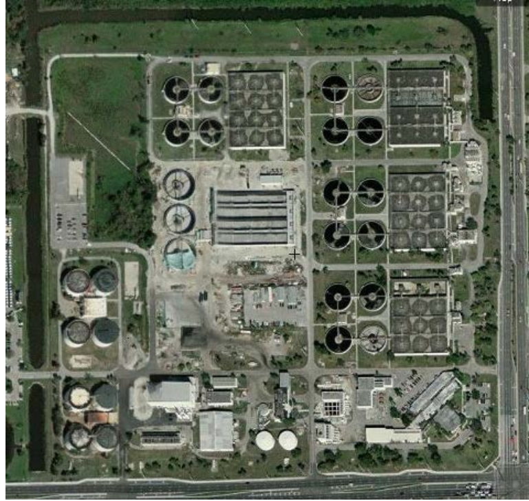
Figure 5: Aerial photograph of the Broward County North Regional Wastewater Treatment plant
