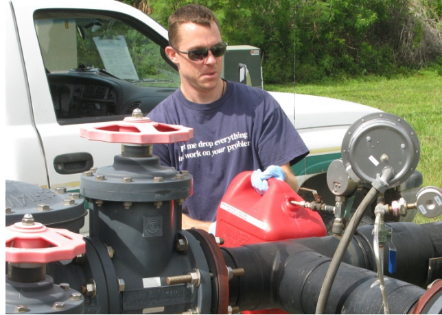
Figure 6: Leachate Sampling on 7/18/2012
